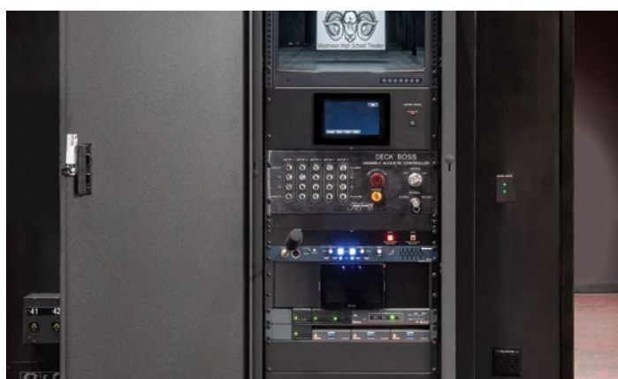
PCD installed a backstage AV rack with a video monitor featuring an audience view of the stage.
