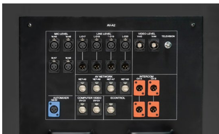
PCD installed panels on all four corners of the backstage area for AV access directly to the control room and PA.
