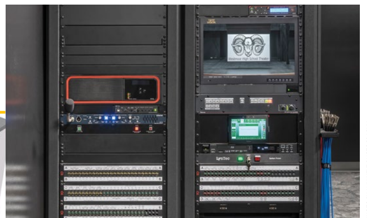
PCD installed an AV rack to control everything from the loudspeaker sound mix to the assisted listening devices
