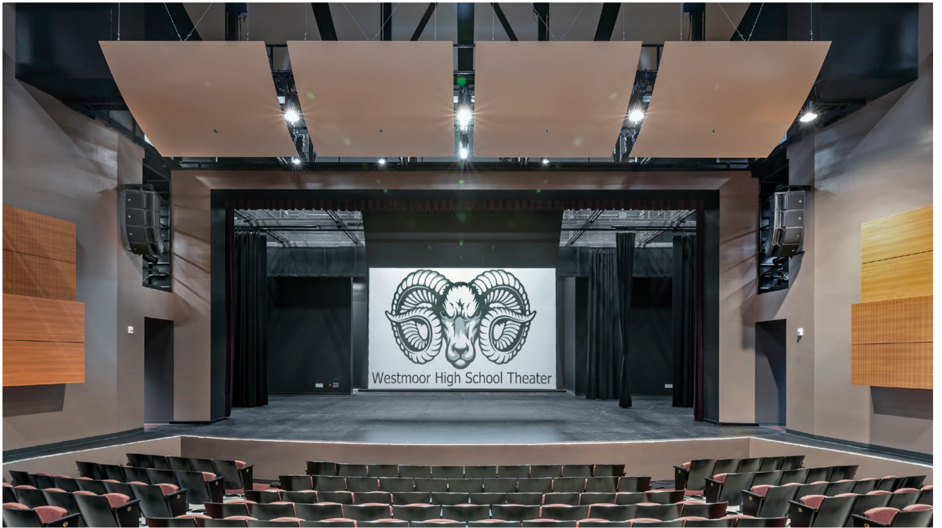
PCD installed a 20-foot wide Draper screen with a rear projector on the stage of the Westmoor Theater.
